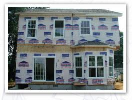
Just before the module goes out the door, the interior is swept clean, it's wrapped tightly in sheets of plastic, and then loaded onto its transport carrier for its trip to the building site.
